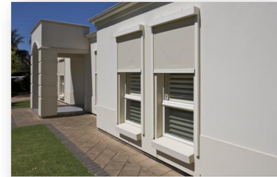
External Window Blinds
